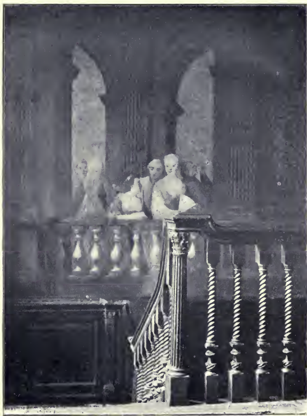
STAIRCASE AT 75 DEAN STREET.
